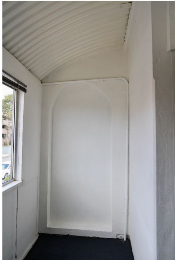
Figure 24 View of the western end of room 9.
