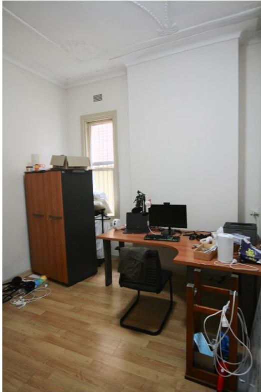
18. View of the second ground floor room.
