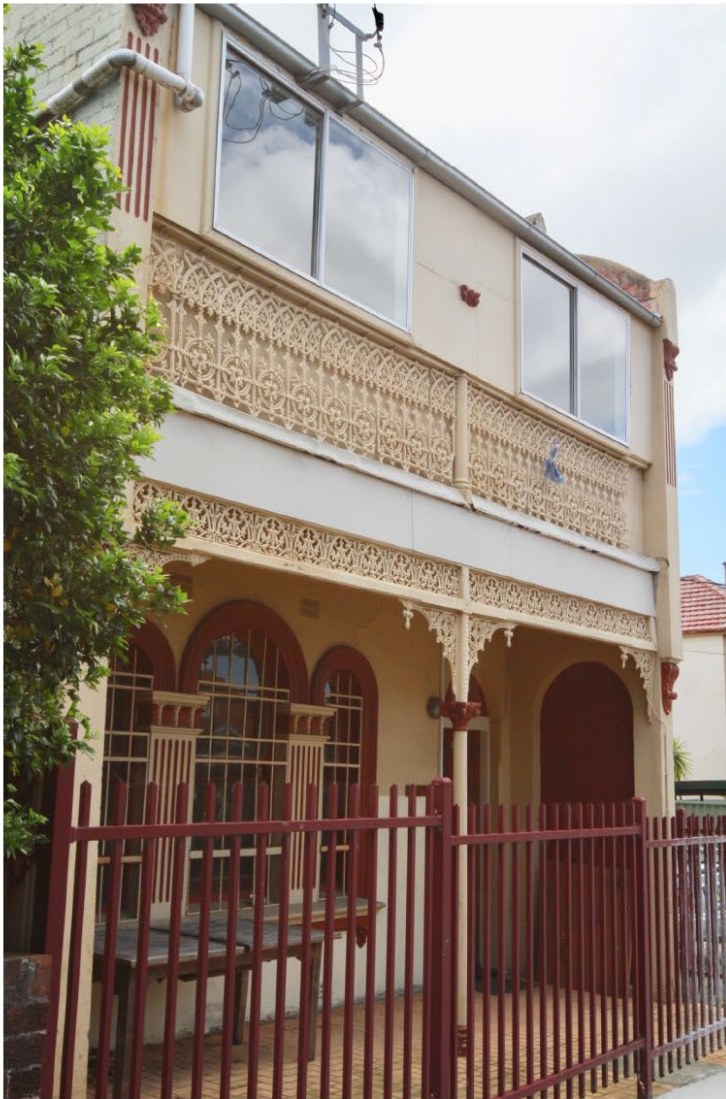
Figure 3. View of the front of the house.
