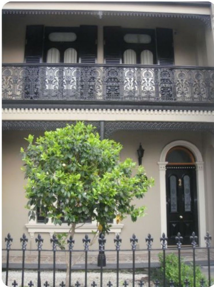
Figure B This photograph shows the model for the timber dentil frieze and timber moulding on the fascia to the verandah beam. It also shows the cast iron first floor frieze. It shows the tiled ground floor verandah with the slate edge.
