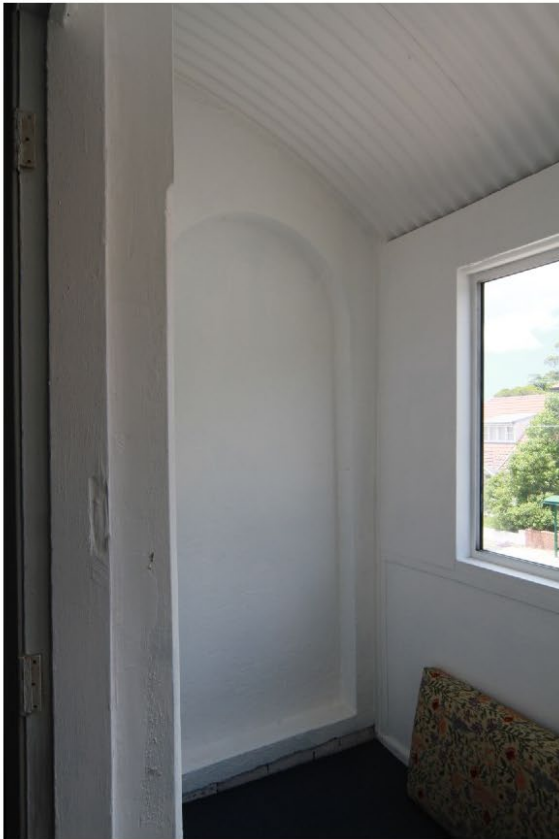
Figure 23 View of the western end of room 9.
