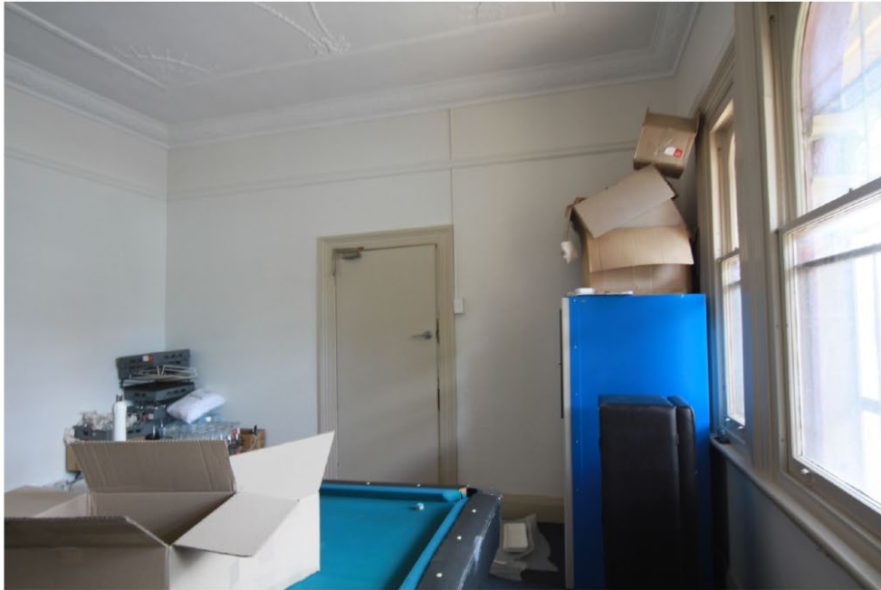
15. View of the ground floor front room. The interiors of the ground floor have been extensively altered and contain very little of the original building fabric. In this room the double hung window and architrave appears to be the only original building fabric.
