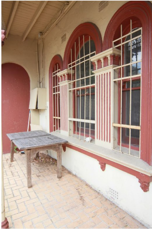
11. View of the ground floor front verandah.
