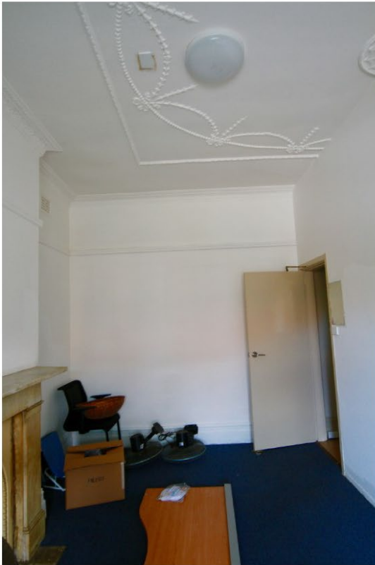
34. View of the front room, which has been subdivided.
