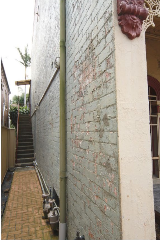
5. The photograph shows the western facade, with the later brick paving and the later external concrete stairs and metal handrail.
