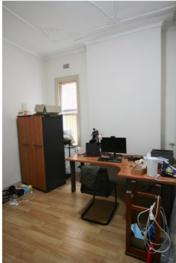
Figure 12 the western wall of Room 2 showing the original chimney breast, double hung window and architrave.
