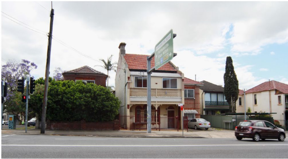
View of the front of No. 37 Liverpool Street in the context of surrounding buildings, viewed from Liverpool Road.
