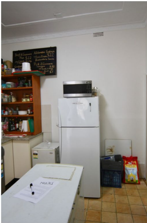
23. View of the ground floor kitchen.
