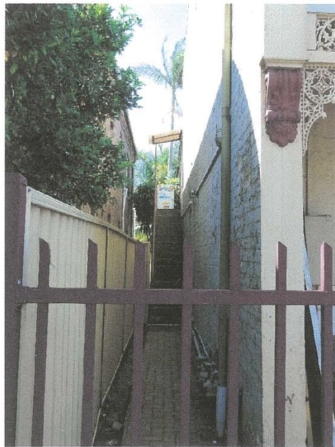
Photograph 3: Subject site, stairs to first floor to be removed.
