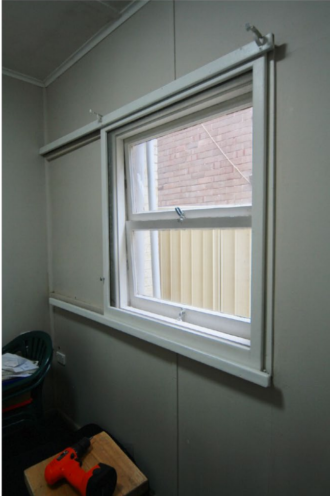
Figure 16. The western wall of space 3.
