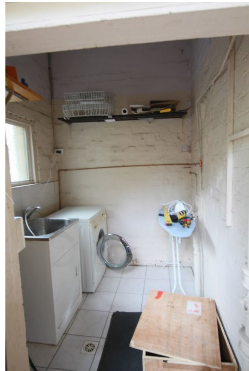
24. View of the ground floor laundry.
