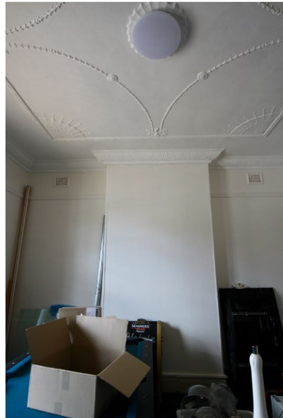
Figure 9. This photograph shows the western wall of the front room in the principal building form of the house and the Inter War ceiling and cornice that replaced the original Victorian ceilings and cornices. Wall vents are later. The mantel and fireplace have been
