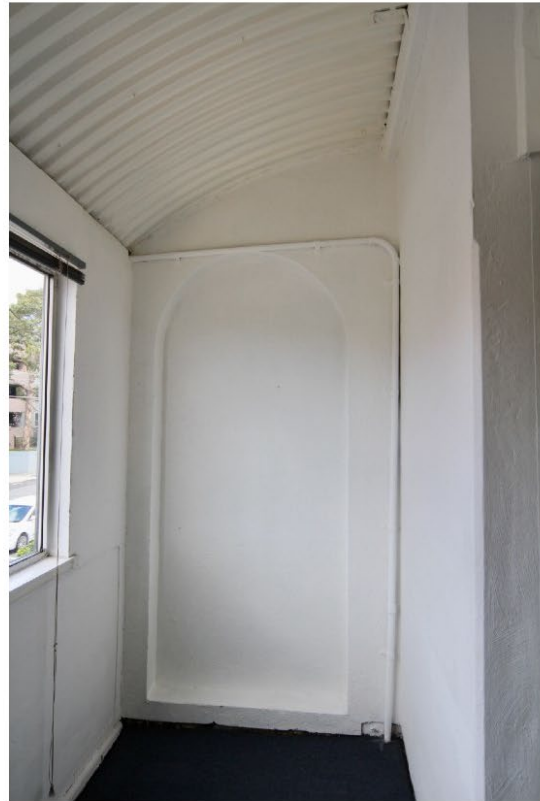
35. View of the infilled front verandah.
