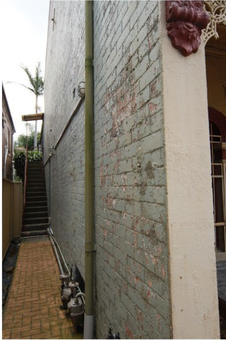
Figure 9. Brick elevation on the western facade.
