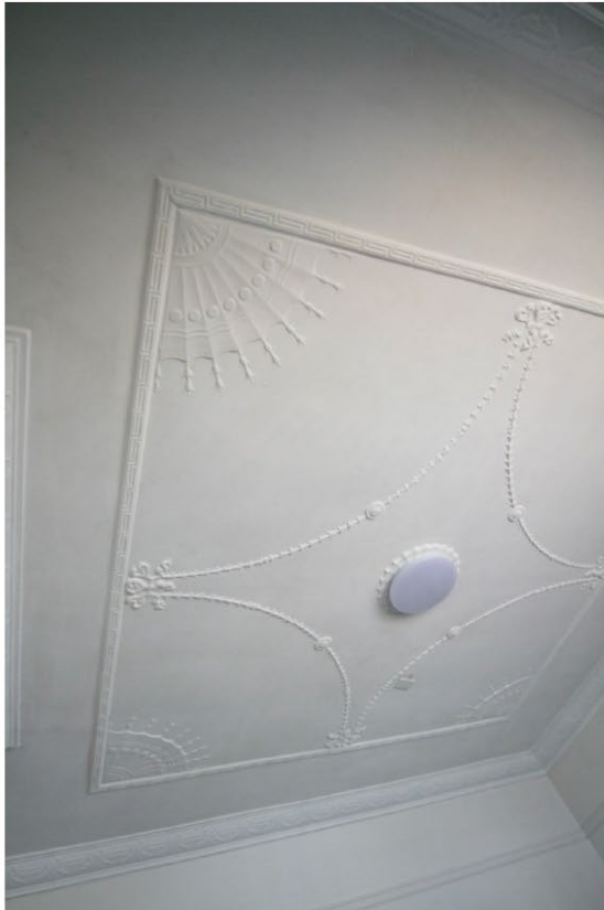
16. This photograph shows that Inter War decorative ceilings and cornices replaced the original Victorian ceilings and cornices.
