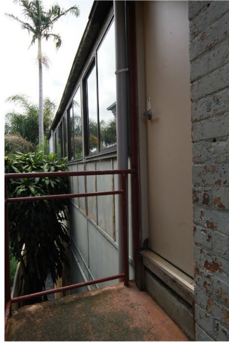
Figure 10 Mid century facade on the western facade.
