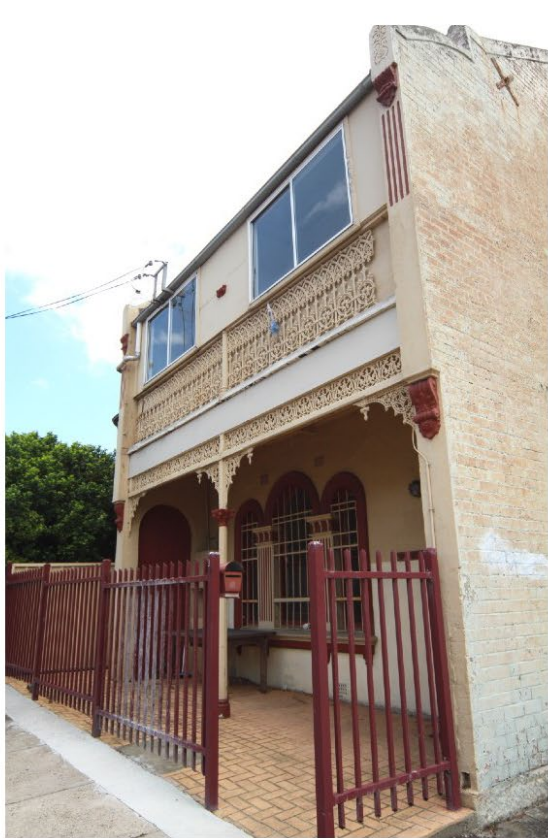
3.View of the front facade showing the later front fence. showing the later additions including the addition of a non original metal front fence and gate, Addition of non original brick paving to the street front zone and verandah, the elimination of the original verandah step down.
