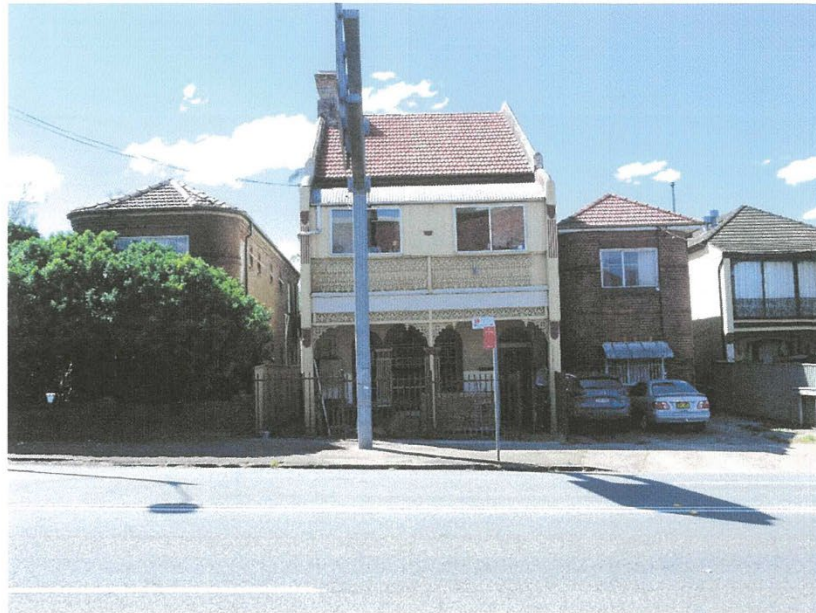
Photograph 1: Subject site, 37 Liverpool Road Ashfield
