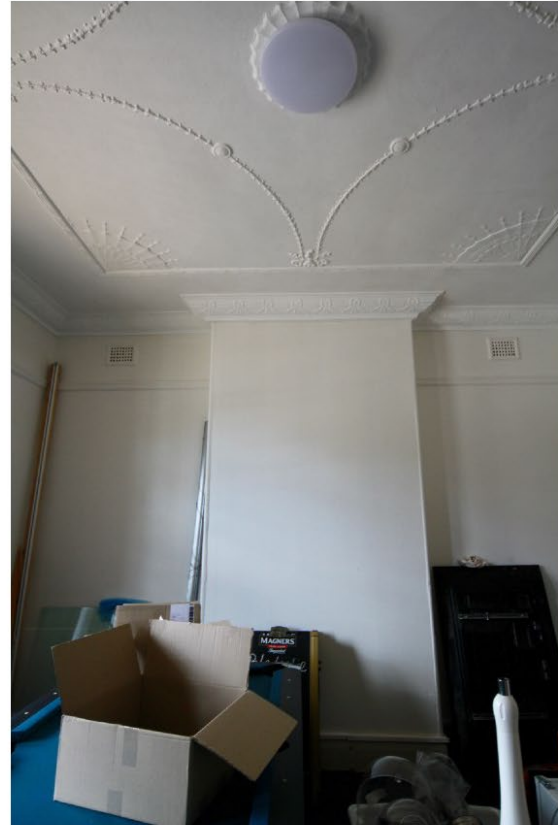
17. This photograph shows the front room in the main section of the house and the Inter War ceiling and cornice that replaced the original Victorian ceilings and cornices. Wall vents are later. The mantel and fireplace have been removed.
