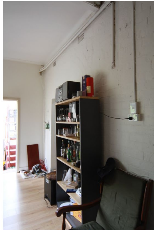
Figure 18. View of Space 7 looking towards the northern wall.
