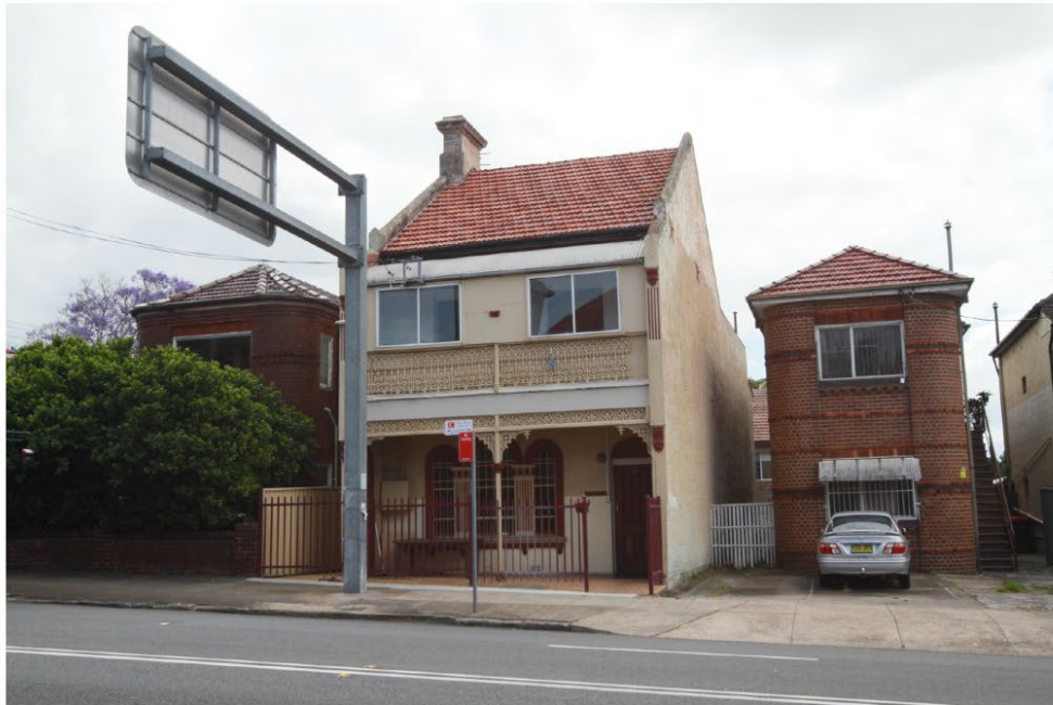
Figure 1. The front of No. 37 Liverpool Road.
