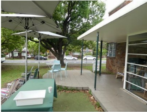
Facing east at the front of the building.
