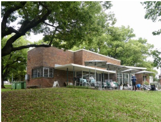
The building from the north-east
