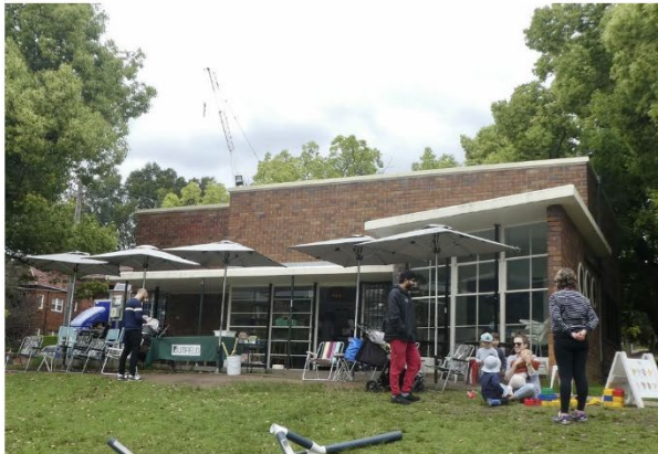
Umbrellas disrupt the main elevation
