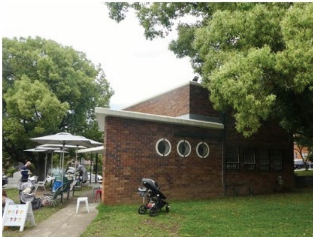
The building from the east
