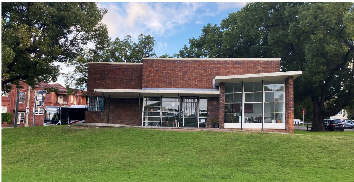
Figure 3: Site photo of existing building taken from Yeo Park.
