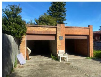
Figure 37: View of the garages and cementitious apron to the rear of the site.
