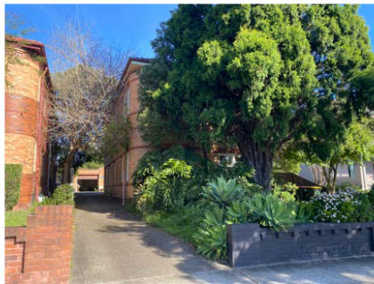
Figure 4: View of the front elevation facing southwest.
