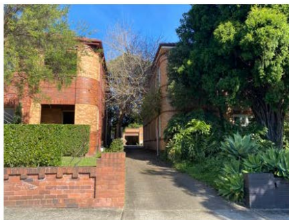
Figure 34: View of the driveway from Hillcrest Avenue along the eastern boundary.
