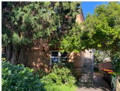
Figure 6: View of the front elevation facing south.
