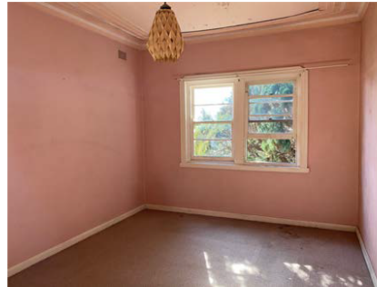
Figure 24: View of Bedroom 1 facing northwest.
