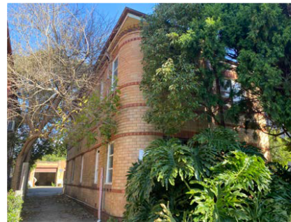
Figure 5: Detailed view of the external brickwork facing south.
