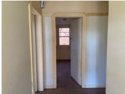
Figure 23: View of the entry hallway facing east.
