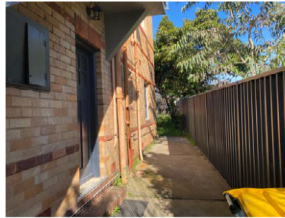
Figure 9: View of the western elevation facing south.
