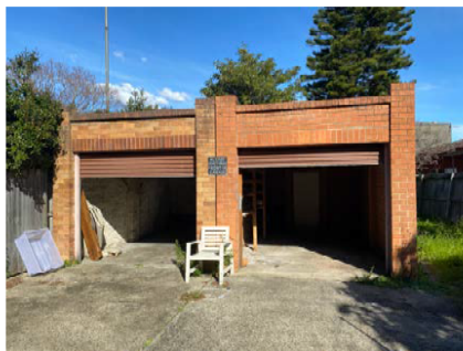
Figure 10: View of the garages at the rear.
