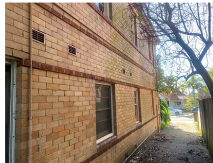
Figure 7: View of the eastern elevation facing north.
