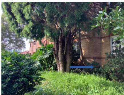
Growing within 3m of the building
