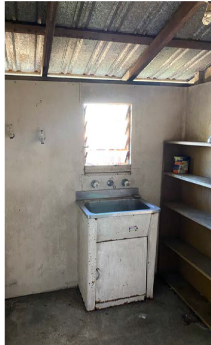
Figure 31: View of laundry facing south.
