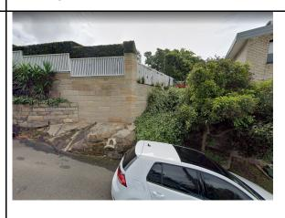
Figure 4: 2020 Google Street view showing the sandstone outcrop with the concrete slab and stairs removed and the sandstone retaining wall to 2-4 Lookes Avenue.
