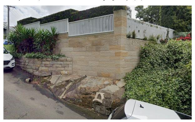
The extent of the sandstone rockface extends to where the sandstone garden bed is located and if the garage door commences at that location, there is concerns of whether the minimum 2200 mm internal heights associated with a garage can be achieved
