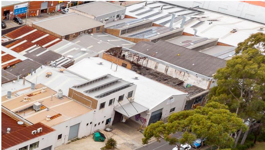
Figure 2: Aerial view of the dilapidated site (Matthew Markakis, 2021)
