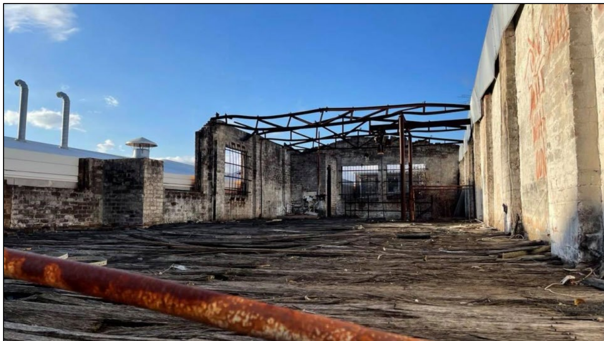
Figure 5: First floor of subject site facing towards the rear (Corona Projects 2021)
