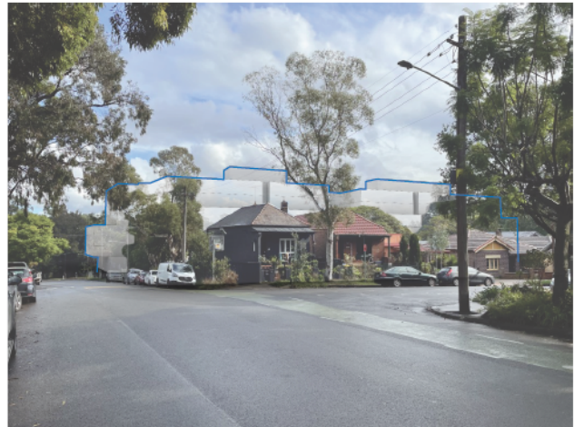
View H - Corner Lords Road / Davies Street
