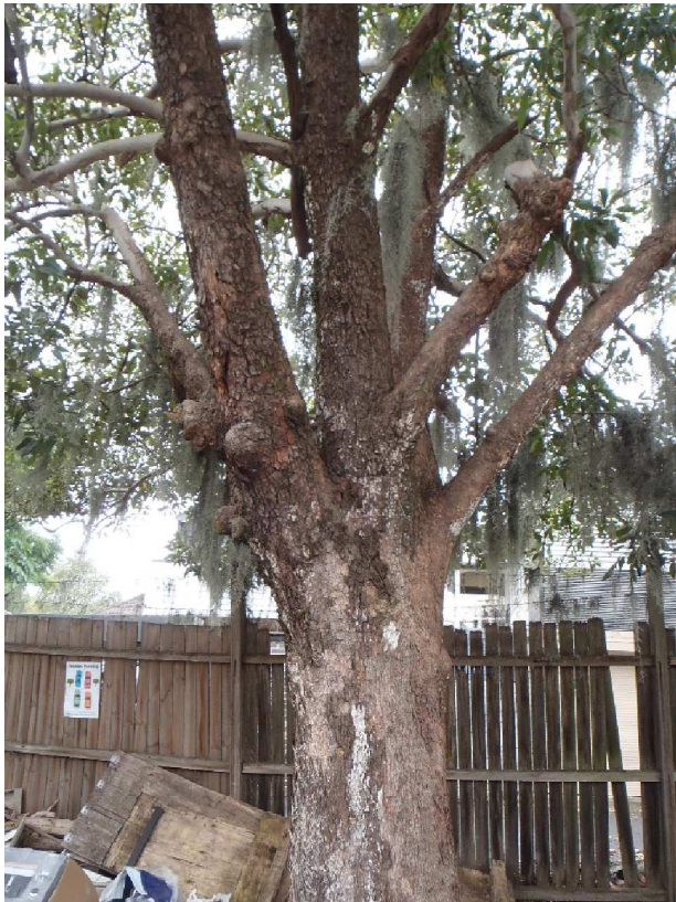
Figure 21. Tree T9. Slight stunting to tree. Rubbish dumped at base. Davies Lane in background. Tillandsia growing on limbs. Fungal mycelia present on trunk. Vertical split in trunk (refer next photo)
