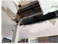
Figure 24: Missing section of plasterboard ceiling in rear room on ground floor.
