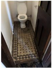
Figure 39: First floor bathroom showing tessellated tiles, skirting and walls, in poor condition.
