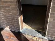
Figure 26: Damaged slate threshold.
