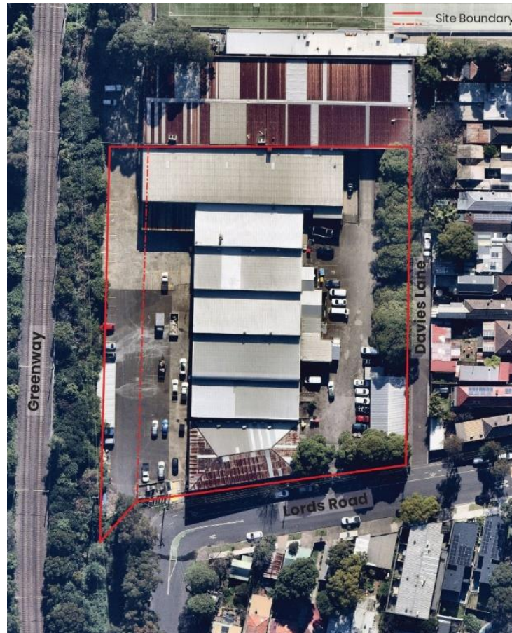
Figure 6: Site area showing building location
