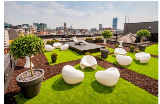
Figure 13: roof gardens help to cool the space and reduce the urban heat island effect.
