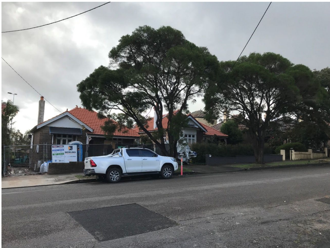
Figure 2 Site Photo – Empire Street frontage
