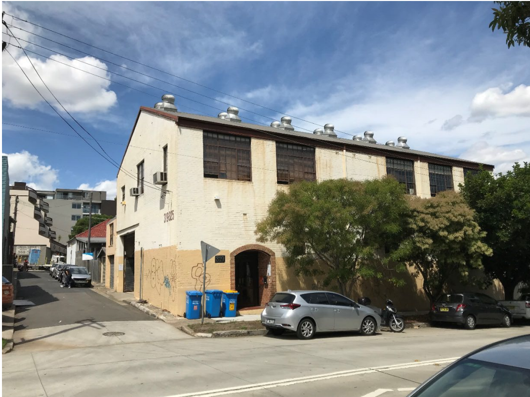
Figure 2: Site viewed from Trafalgar Street
