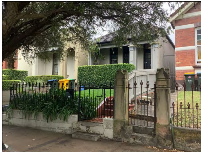
Figure 32: Showing the relationship of No. 143 Annandale Street to its neighbours to either side.
