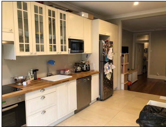
Figure 27: The kitchen looking back towards the dining room. Note the plasterboard ceiling and quad cornice and the modern fit out and finishes.
