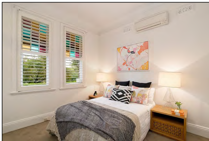
Figure 19: Bedroom 1, showing the coloured panes to the double hung sash windows, the profiled timber architraves, skirting boards and picture rails. Note the decorative wall vents.
