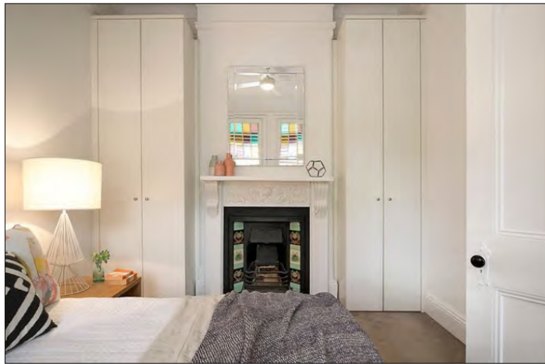
Figure 20: Bedroom 1 showing the fireplace with timber mantelpiece and inset tiles within the cast iron coal grate. Note also the four panel door.
