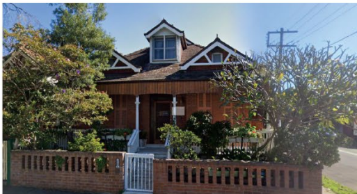
No. 22 a Bungalow style house dressed in motifs without regard for accurate rendition. Additions of a minor scale are obtrusive in the streetscape context: timber valance, aluminium framed windows, louvre shutters and fencing not appropriate to the building typology. Breaks the cohesiveness of materiality.
