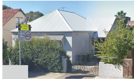
No. 9 Post war Austere dwelling. Its envelope swathed in grey paint and matching grey corrugated iron awnings, stripped of its original finish and lack of original detailing.
