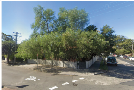
No. 13 corner sited dwelling is totally obscured by plantings and trees. The screen of vegetation breaks the streetscape pattern, rhythm and texture.
