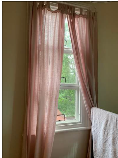
Figure 53: Window in the southern wall with original architraves and later awning sashes. It is proposed to replace the sashes with timber framed double hung windows. Figure 54: Door in the western wall. Later door panel with original architraves and blocked in fanlight. It is proposed to remove this door.
