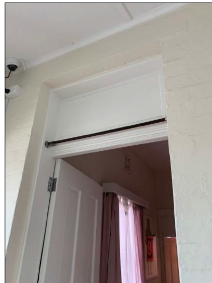
Figure 50: Later door panel into Room 3 with replaced/modified architraves. It is proposed to remove this door and widen the opening.
