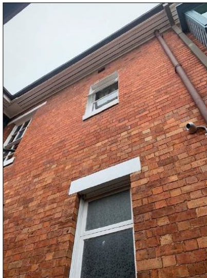
Figure 18: Looking up towards the first floor window with two awning sashes fitted.
