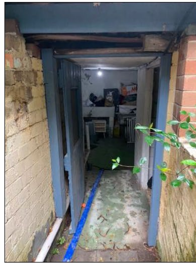
Figure 23: Looking east into the passage way into the basement rooms from the rear yard. The door is a ledged and braced timber door with central glazed panel.
