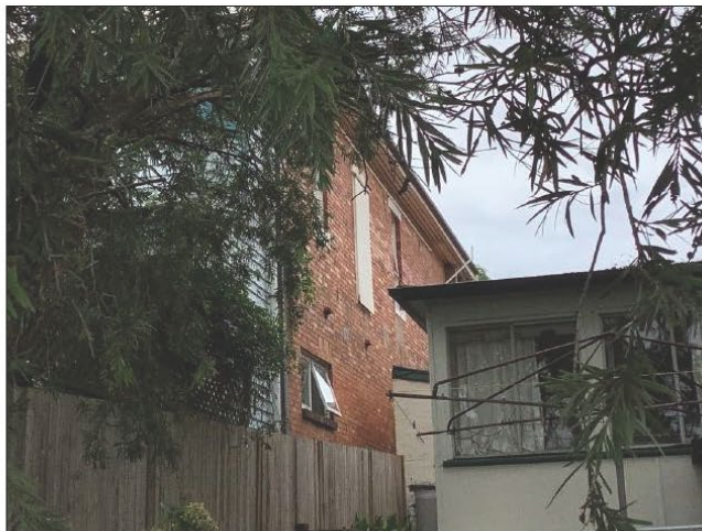
Figure 10: Later brickwork and window at first floor level in the southern elevation. Note also the slatted eaves.
