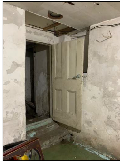
Figure 30: Cut down four panel door between the laundry and the larger store room. Figure 31: Vent in the northern wall of the larger store room.
