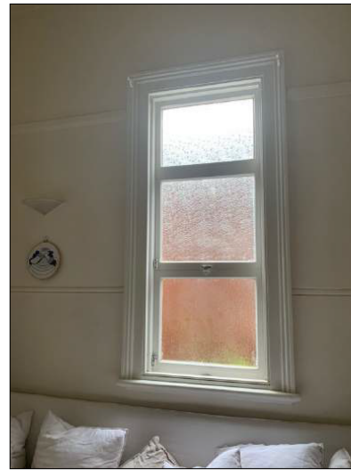
Figure 34: Window in the northern wall, also showing the indented line in the plaster and the later picture rail.
