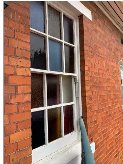
Figure 16: Ground floor window on the northern side that has been replaced with three awning sashes.
