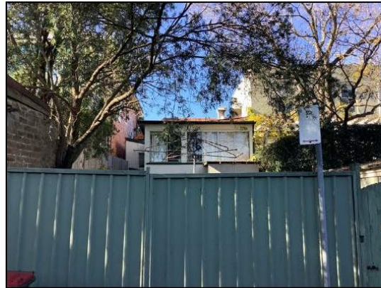
Figure 64: The rear of No. 340 Annandale Street from Breillat Lane.
