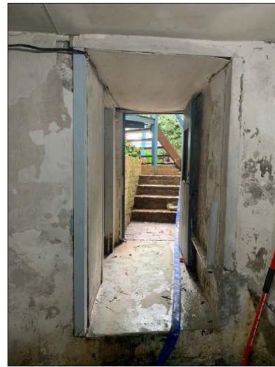
Figure 23: Looking east into the passage way into the basement rooms from the rear yard. The door is a ledged and braced timber door with central glazed panel.
