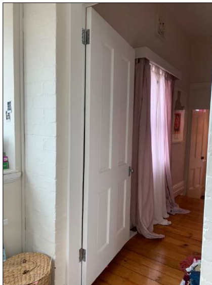
Figure 50: Later door panel into Room 3 with replaced/modified architraves. It is proposed to remove this door and widen the opening.
