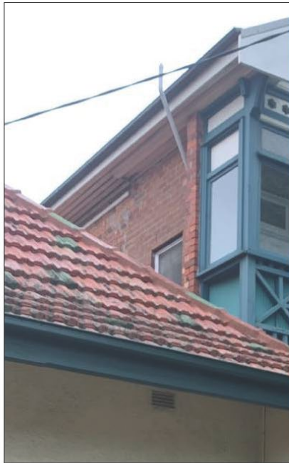
Figure 10: Later brickwork and window at first floor level in the southern elevation. Note also the slatted eaves.
