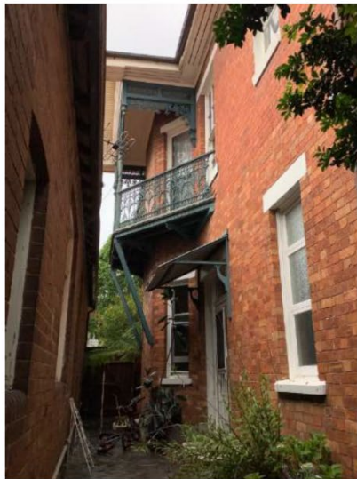
Figure 12: Looking east along the northern elevation.
