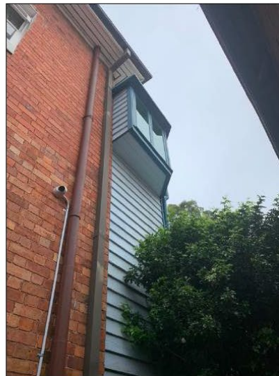
Figure 18: Looking up towards the first floor window with two awning sashes fitted.
