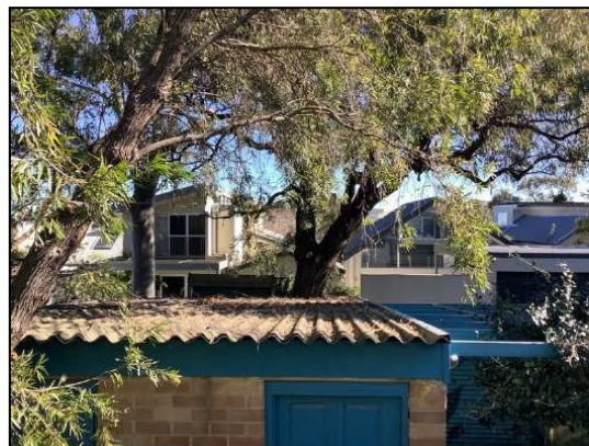
Figure 66: Rear of the dwellings on the opposite side of the lane. Note the lack of consistency in form and pattern of openings.
