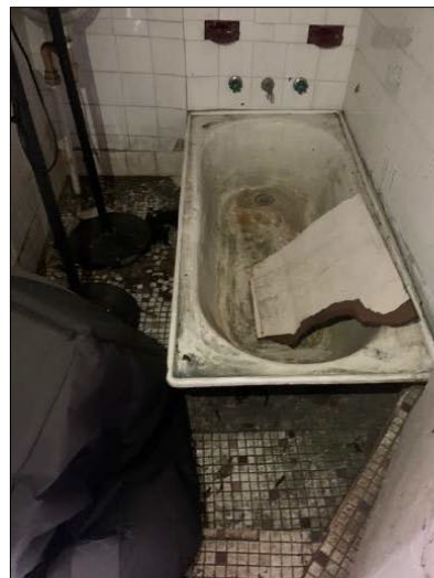
Figure 25: Post World War II bathroom fit out.
