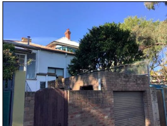
Figure 65: The rear of No. 342a Annandale Street from Breillat Lane.
