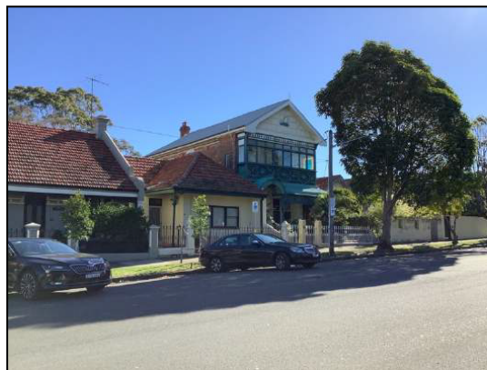
Figure 70: View when closer to the site on approach from the south.
