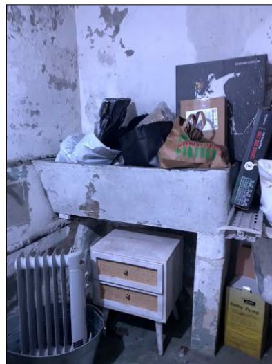
Figure 28: Eastern wall and the laundry with concrete tub.
