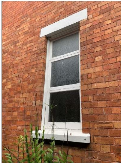
Figure 16: Ground floor window on the northern side that has been replaced with three awning sashes.
