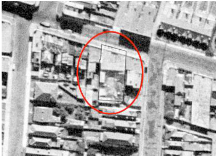
Figure 2.5 Detail from aerial photography dated 1943
