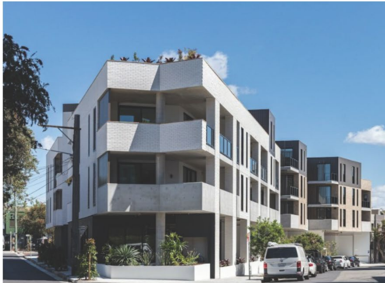
Figure 1: Existing building at corner of Wilford and Gladstone Streets (Nordon Jago Architects)
