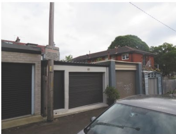
Facing north-west in the lane: part view of rear of No. 41; 43 (centre), 45, 47; home units at No. 49 beyond
