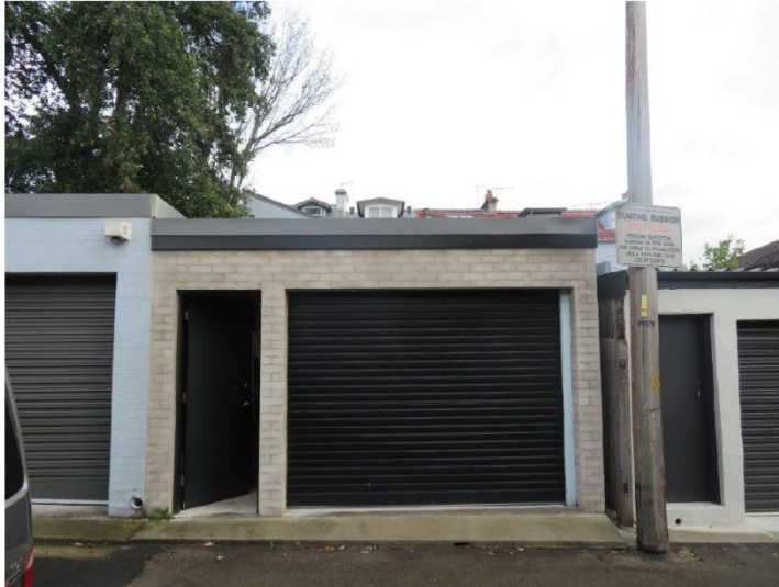
Figure 2: Existing rear garage outbuilding upon laneway
