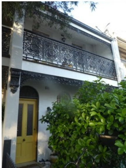
No. 41 from the front gate
