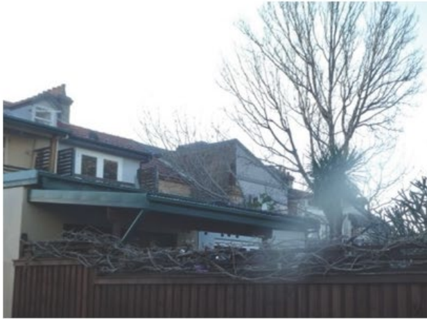
Rear extensions seen from lane to south of No. 33
