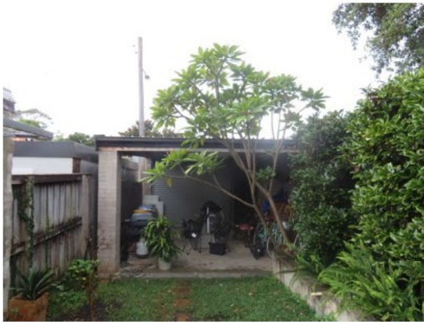
Rear of carport
