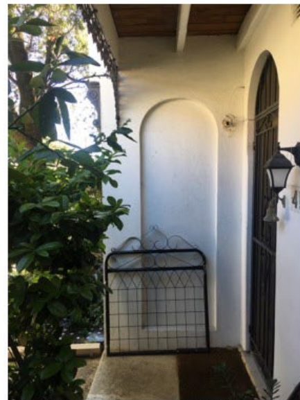
Ground floor veranda with recessed arch
