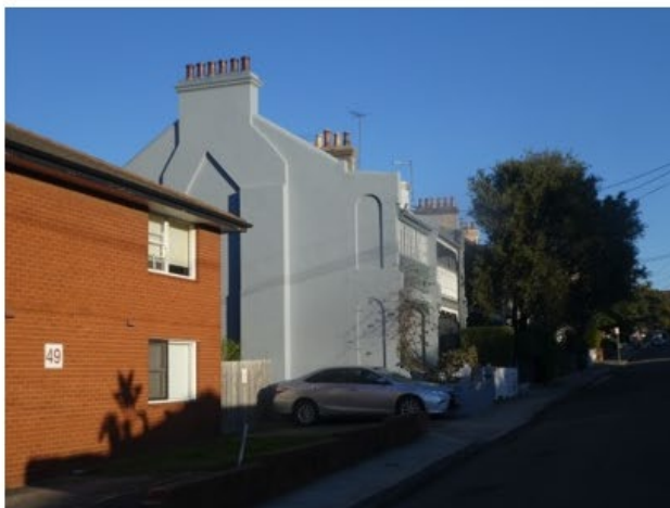
Red brick units extend over site of former demolished terrace house at No. 49, with end wall of No. 47 beyond
