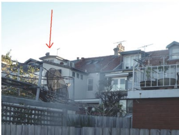
The varied rear extensions to the terrace row with No. 41 arrowed
