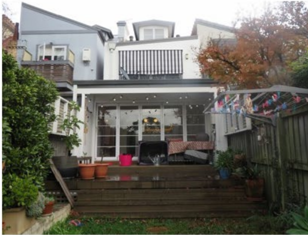
Rear of the house with recent dormer and extensions. Neighbouring houses also extended.
