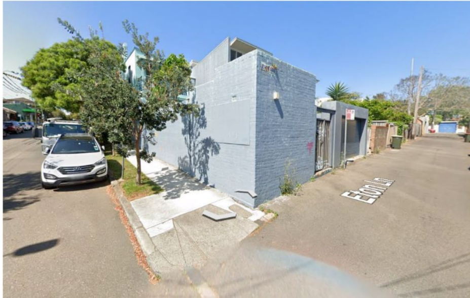
Figure 4 - Photograph of subject property as viewed from intersection Australia Street and Eton Lane
