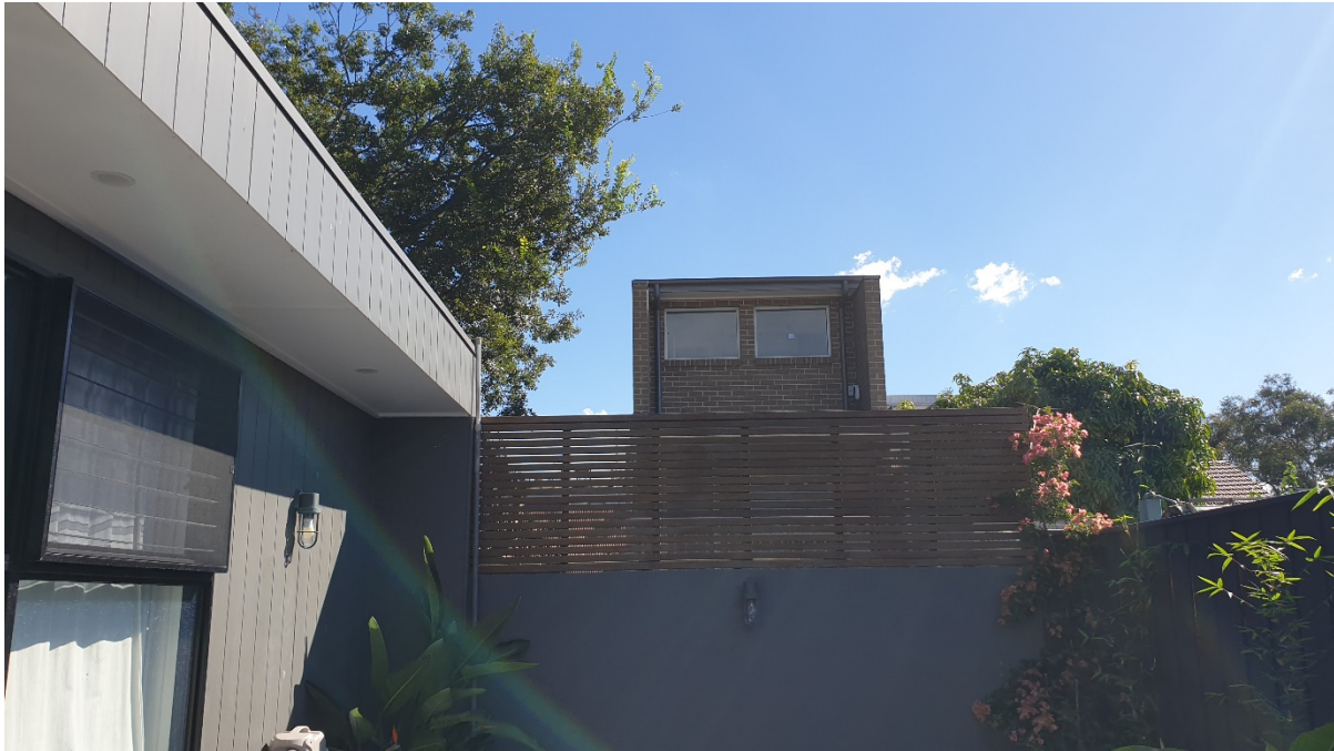
View from the rear private open space of No. 4 Arthur Street
