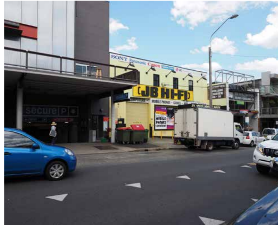
The eastern edge of Norton Street is characterised by large blocks, poor built form and low footpath amenity with many driveway entries.
