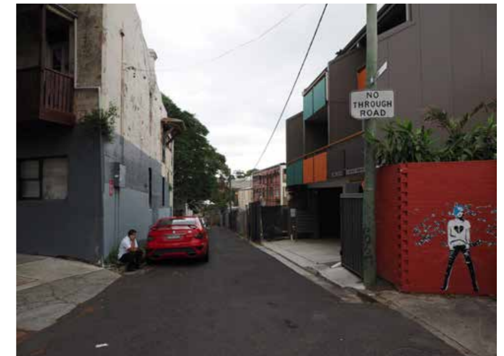
A recent example of residential development fronting McCarthy Lane, behind the Annandale Hotel.
