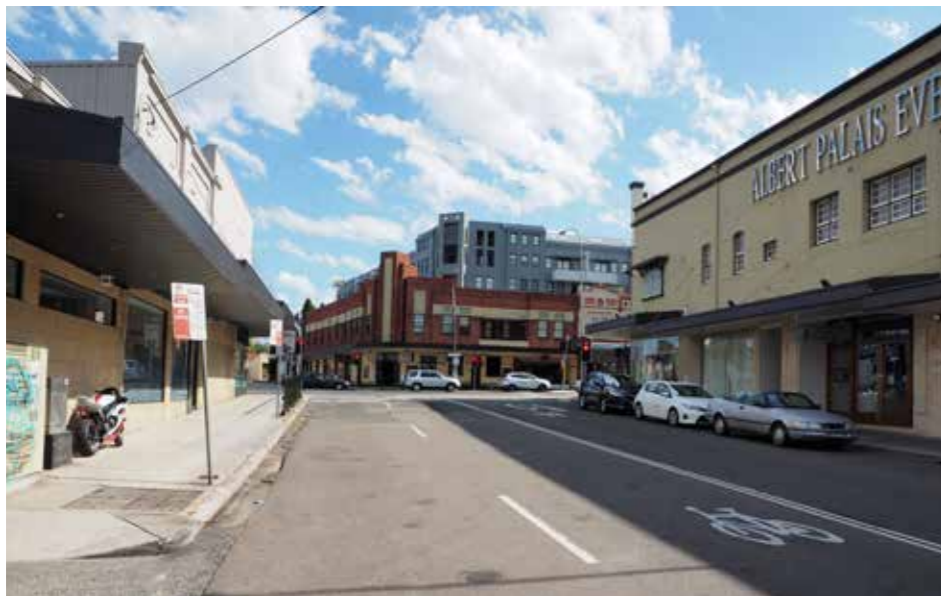
Catherine Street is anchored by the heritage listed Albert Palais Events, but has little greenery or shade. The development on the south side of Parramatta Road illustrates new built form set back from the heritage 2 storey building.
