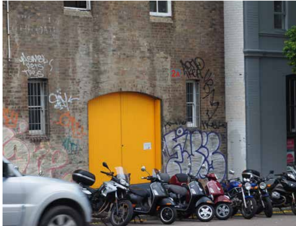
Existing warehouse buildings provide a strong character and opportunity for redevelopment.
