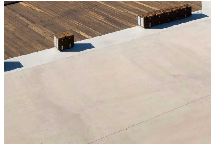
Insitu concrete paving
