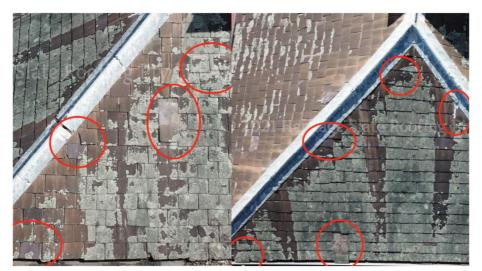
Figure 1 – Location of defects on the existing slate roof (Corona Projects 2021)
