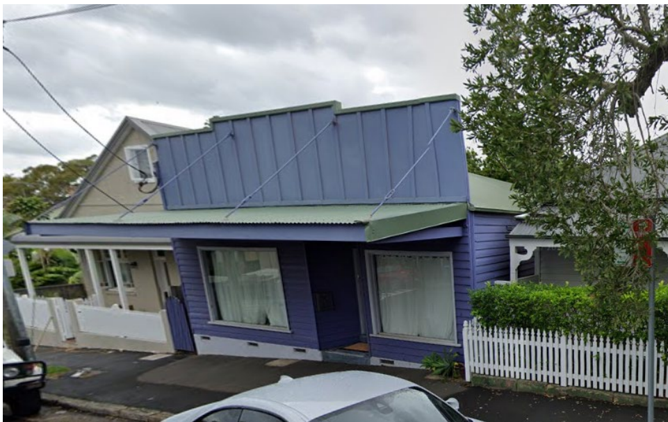
Figure 5: View of No. 174 Evans Street
