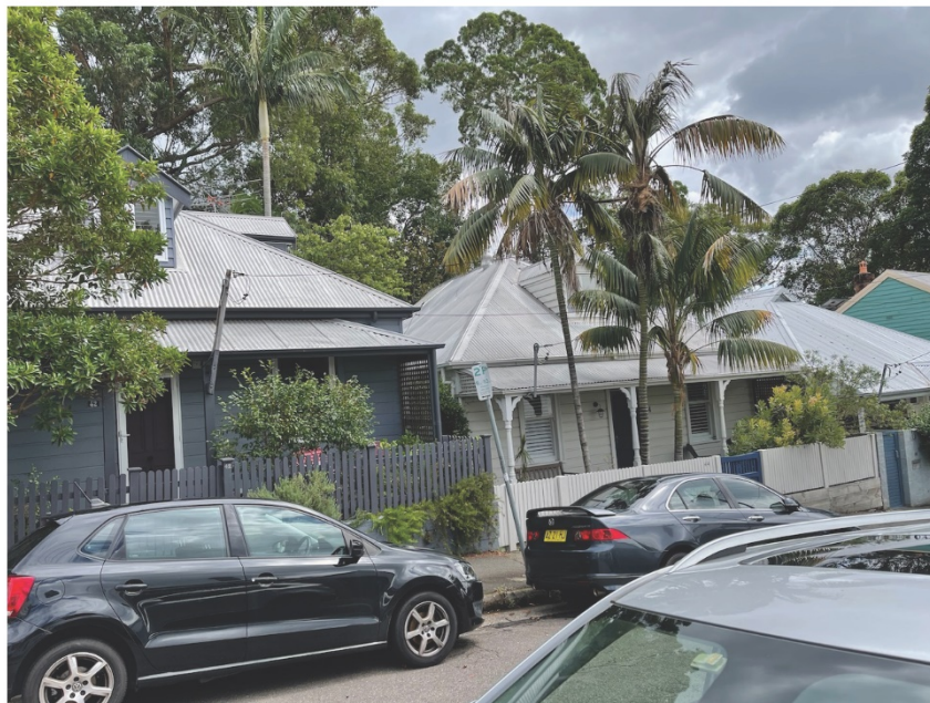
Subject building (red arrow) with 44 College street on the right.
