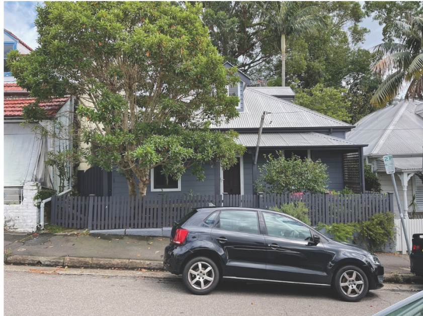
Subject site from College Street, facing north.
