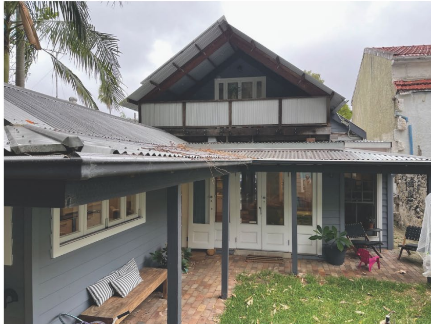
View to rear of the subejct building.
