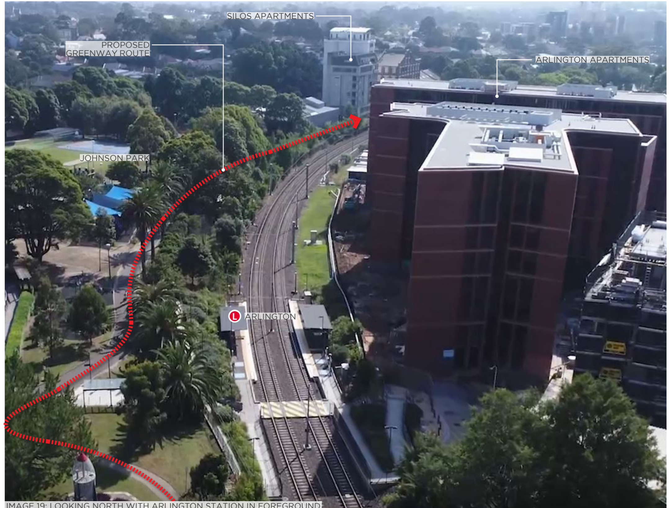
IMAGE 19: LOOKING NORTH WITH ARLINGTON STATION IN FOREGROUND
