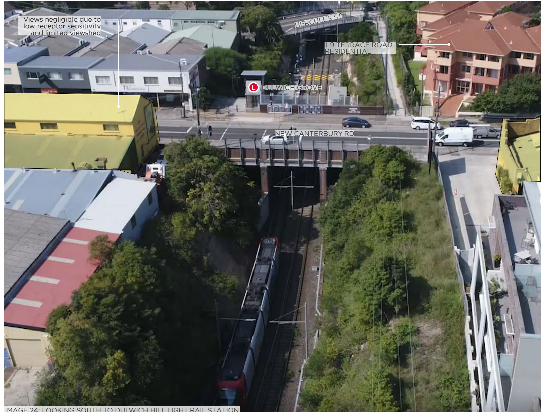
IMAGE 24: LOOKING SOUTH TO DULWICH HILL LIGHT RAIL STATION
