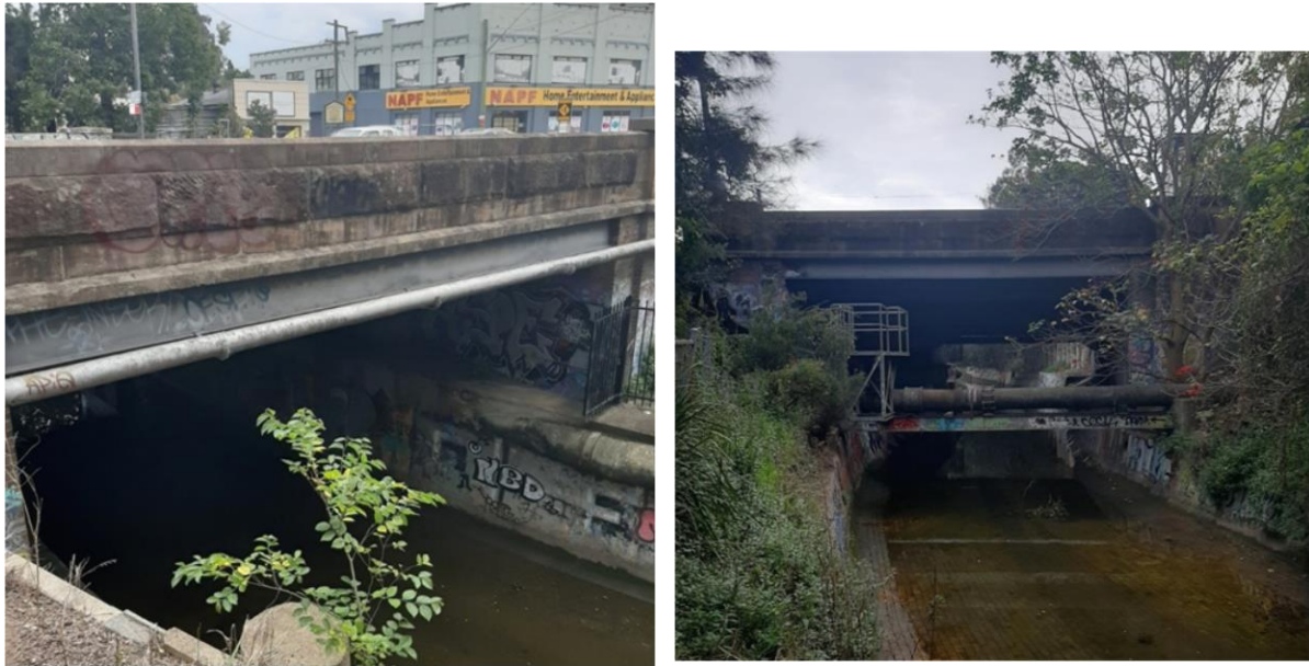
Figure 21: Parramatta Road bridge over Hawthorne Canal containing potential microbat roosting habitat
