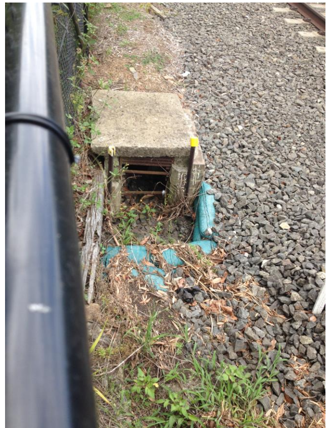
Figure 30: Existing pit inlet downstream of Terry Road
