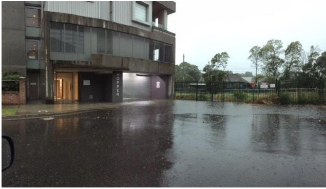
Figure 28: Nuisance flooding at the downstream end of Terry Road
