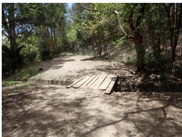
Figure 22: Northern drainage channel in Gadigal Reserve
