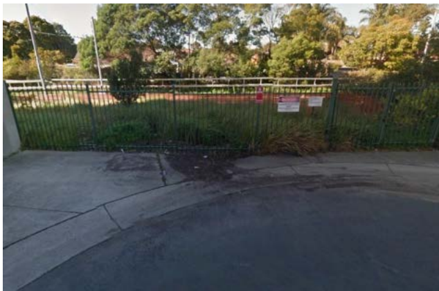
Figure 34: Evidence of blockage at the end of Terry Road
