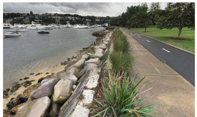
Figure 19: Upgraded seawall at Pearl Bay, NSW
