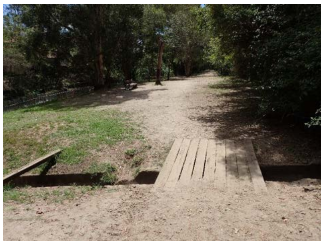
Figure 21: Southern drainage channel in Gadigal Reserve
