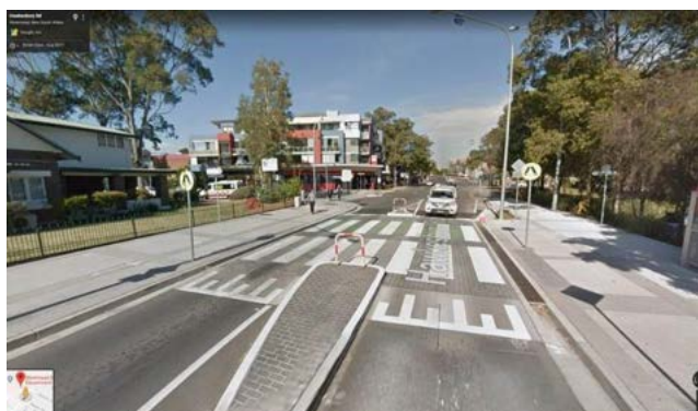
Figure 13: Example of a shared pedestrian and bike crossing at Hawkesbury Road, Westmead
