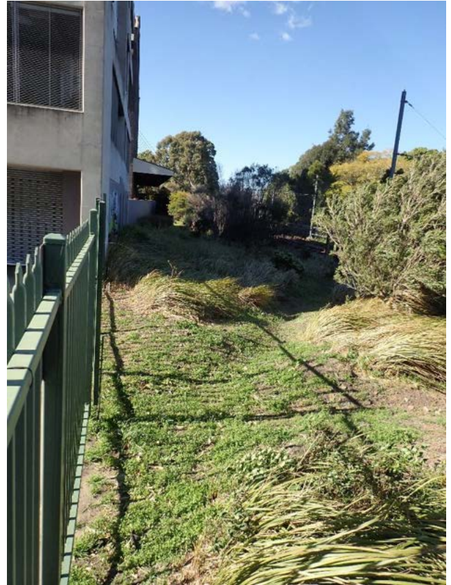
Figure 29: Existing swale downstream of Terry Road (estimated Manning's n = 0.03 )
