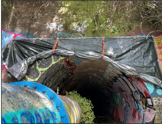
Figure 2: Installed exclusion device prior to lowering
