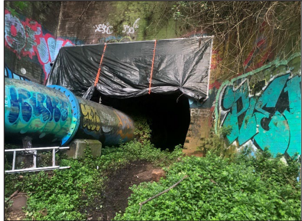
Figure 3: Exclusion Device 40% closed
