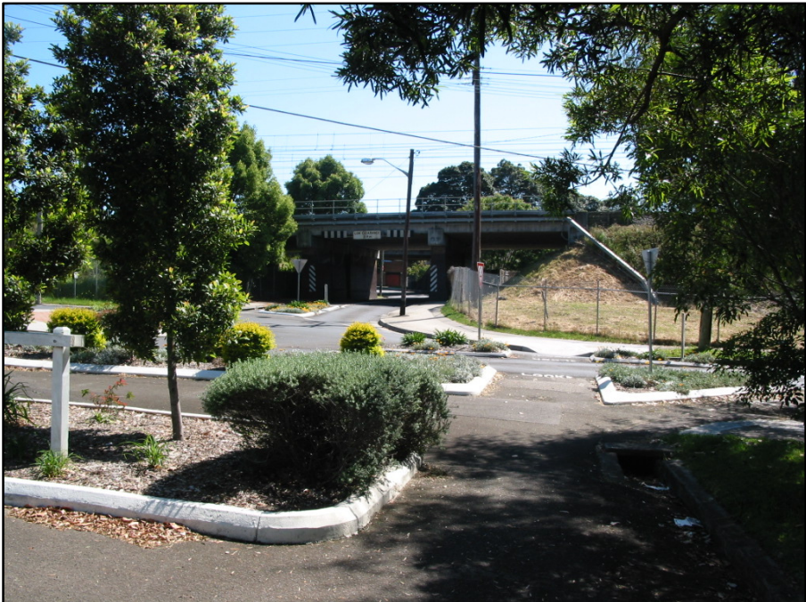
Figure 5-7: Ness Ave underpass
