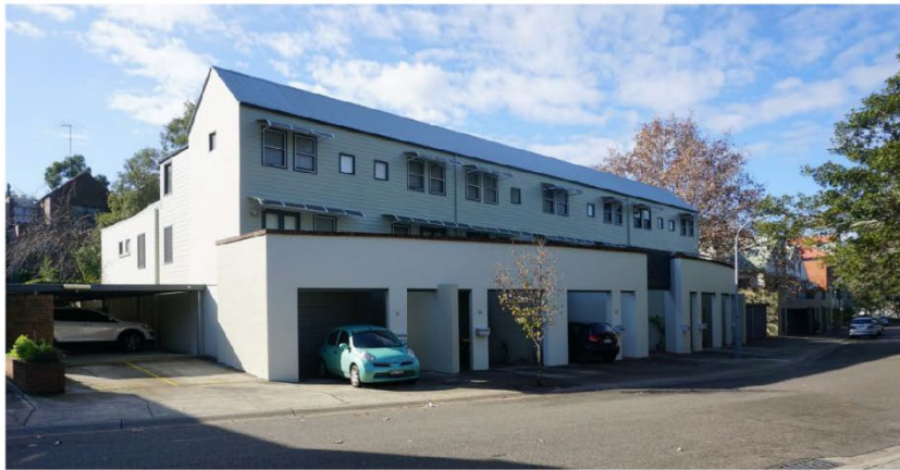
Fig 1: View of 15-27 McKell St Birchgrove
