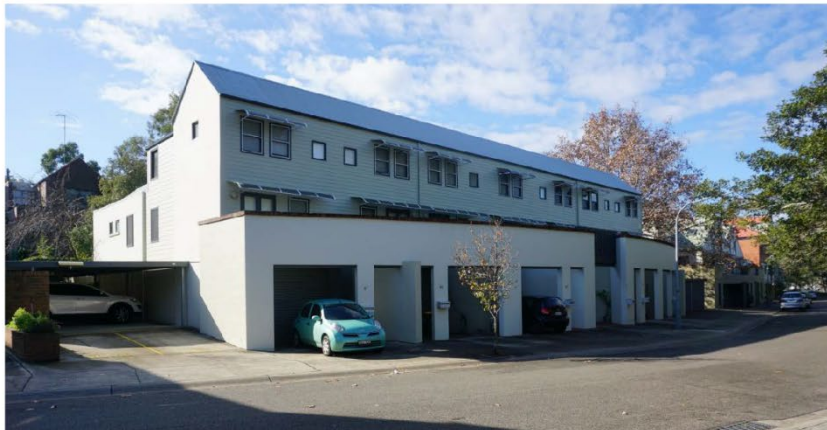
Fig 1: View of 15-27 McKell St Birchgrove
