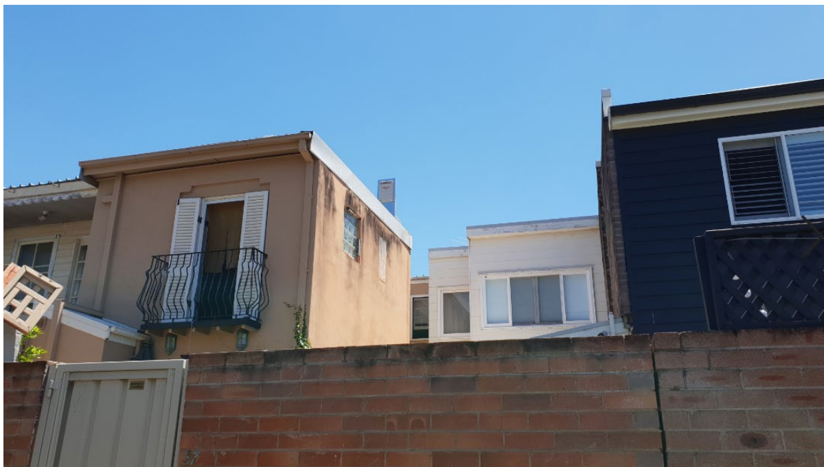
View of the subject site from the rear lane
