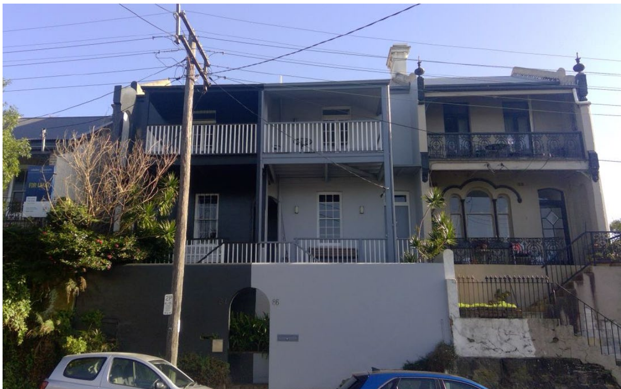
Photo 1: View from Rowntree Street, No.86 is the middle building (light grey)
