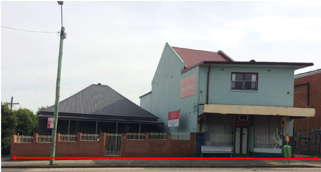
Figure 1: Site viewed from Canterbury Road.
