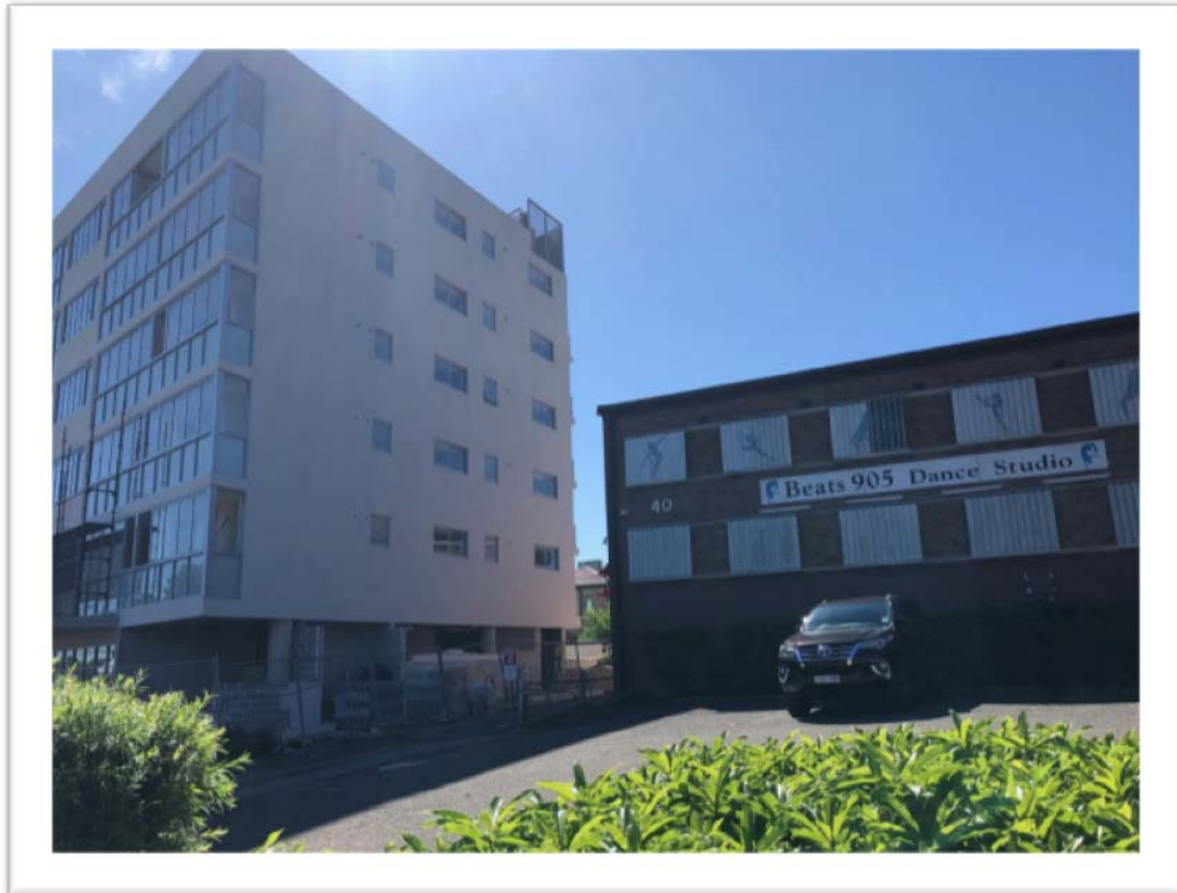
Figure 2 – Site Photo, Southern Elevation of 380 Liverpool Road.
