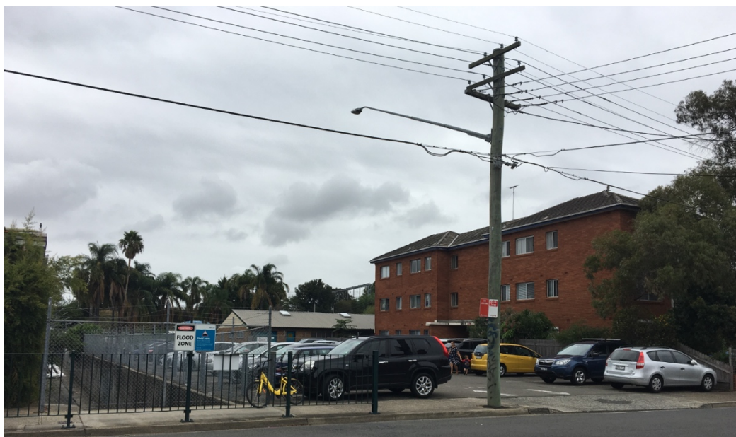
Figure 2 Residential flat building at No. 182 Elizabeth Street
