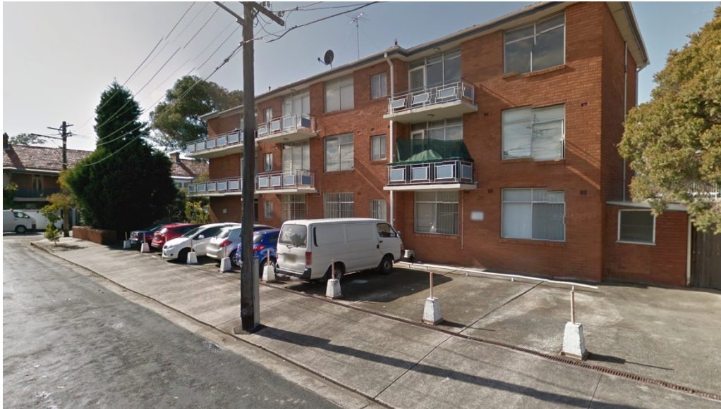
Figure 3 Bastable Street frontage of No. 182 Elizabeth Street
