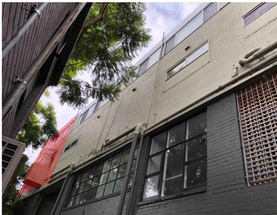
Southern façade from Right of Way (subject lot in red)
