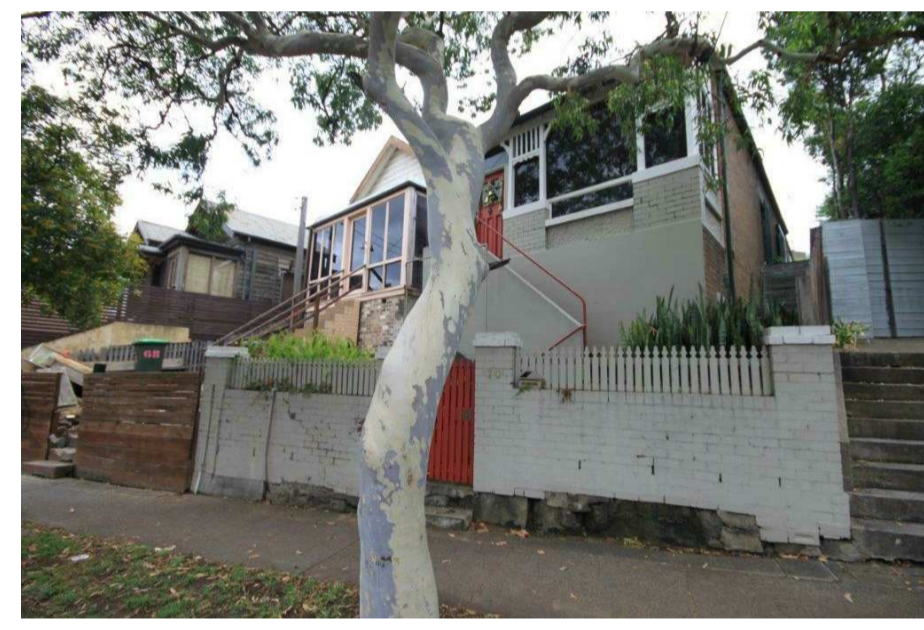
P2 PHOTOGRAPH OF 68-70 BRENNAN STREET
