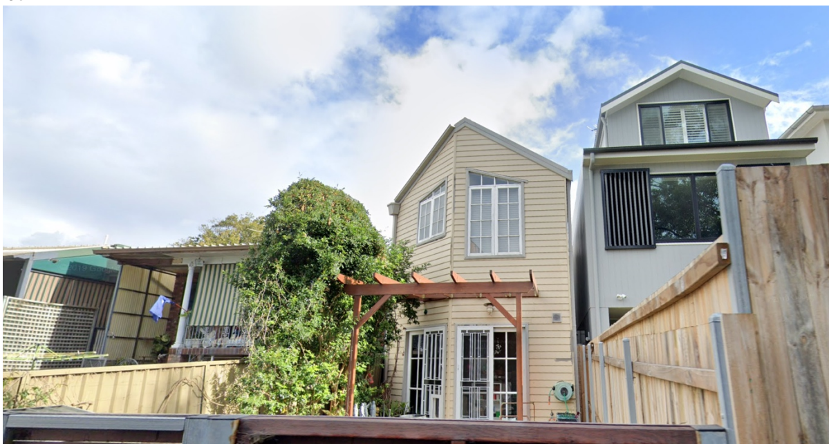
Figure 1: Views of Nos. 20, 22 & 24 Carrington Street from the rear lane facing towards the west.
