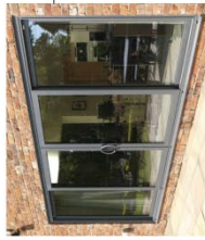
POWDERCOATED ALUMINIUM WINDOWS & DOORS TO MATCH EXISTING
