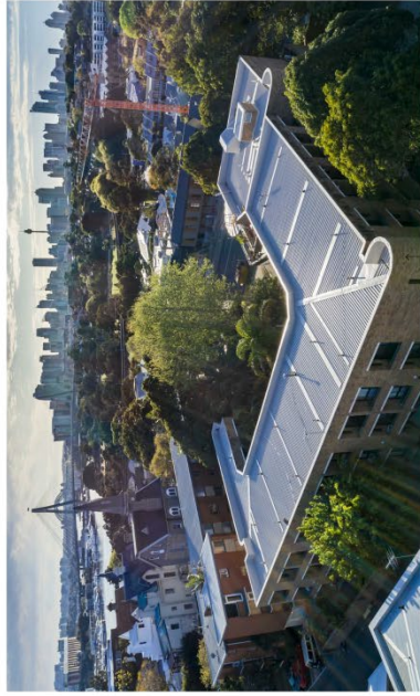
PROPOSED JOHNSTON STREET BALCONIES, MIMIC FRONT FORTH FORM OF THE EXISTING BUILDING FABRIC
