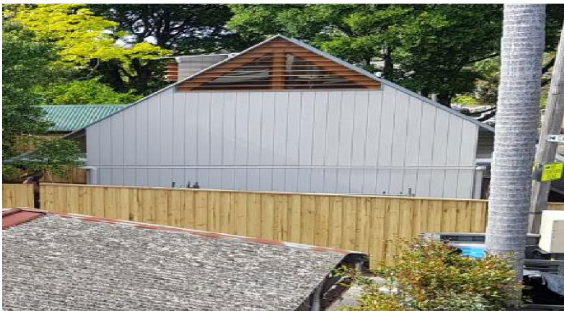
Image 1. First floor storage loft window of 5 Justin Street
