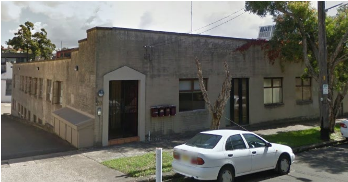
Figure 1: The subject site from Francis Street
