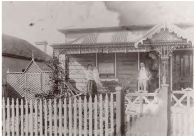
Figure 2.6 An early photo of 82 Moonbie Street, showing the original iron roof and chimney, painted striped verandah roof, filigree iron work and a central gable with lattice (now removed), a screened side fence and the original timber picket front fence and gate. The house name "Glencoe" is just visible and the cast iron lace is picked out in different colours
