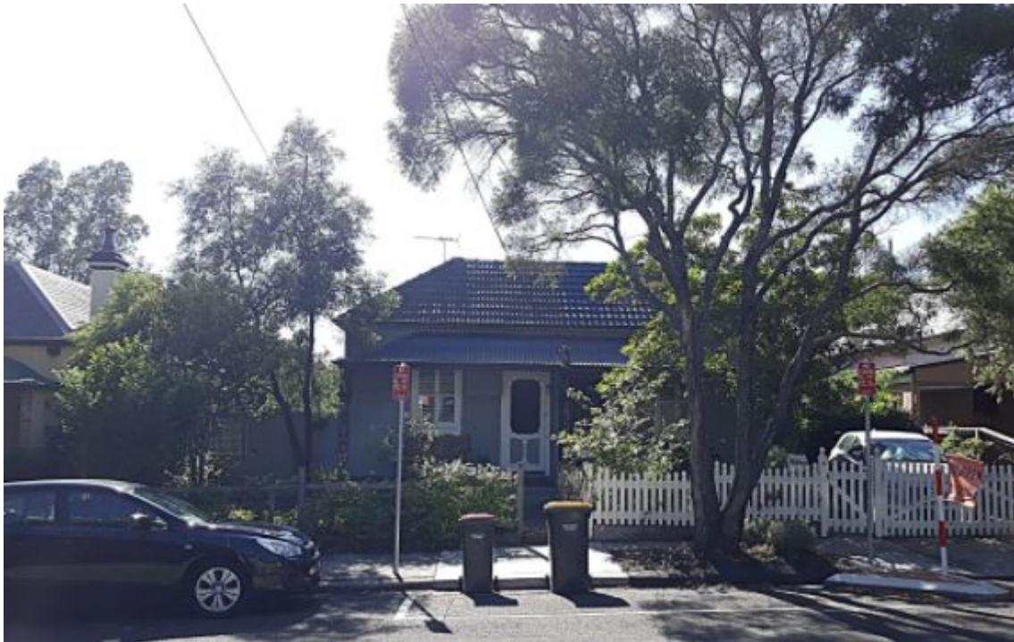
Image 1: View of the site from Moonbie Street
