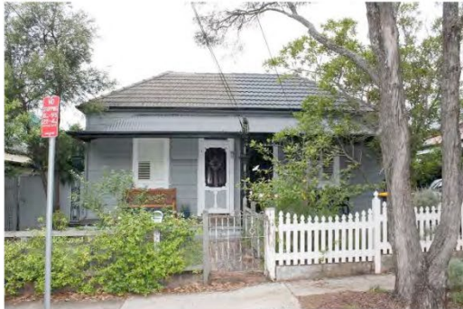
Figure 3.2 82 Moonbie Street Front facade
