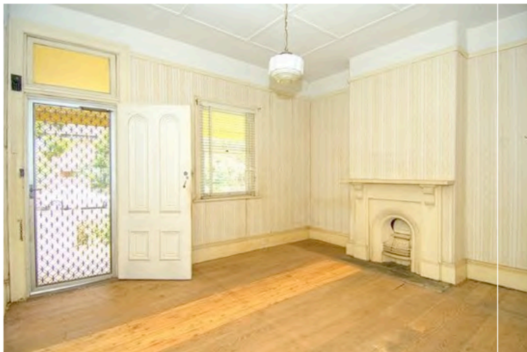
Figure 2.8 View of the front living room in 2007, showing later wallpaper, venetian blind and light fitting. The floorboards have been patched and the fire surround painted. These works may have been undertaken by Meite McGregor in 1955 when she inherited the house following the deaths of her parents
