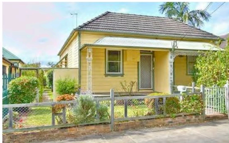
Figure 2.7 82 Moonbie Street in 2007, when it was advertised for sale for the first time in nearly 100 years. By this time the verandah details have been simplified, the gable, lacework and the front chimney have been removed
