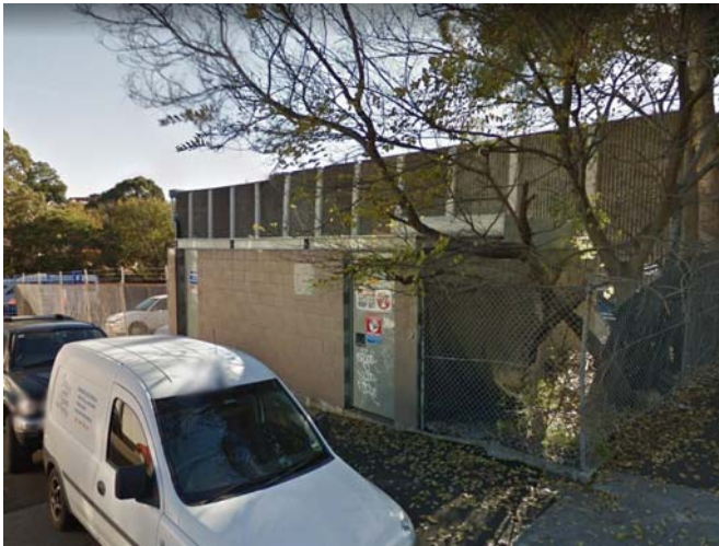
Figure 7 - Kennards Storage Warehouse at 1 - 19 Booth Street opposite the subject site
