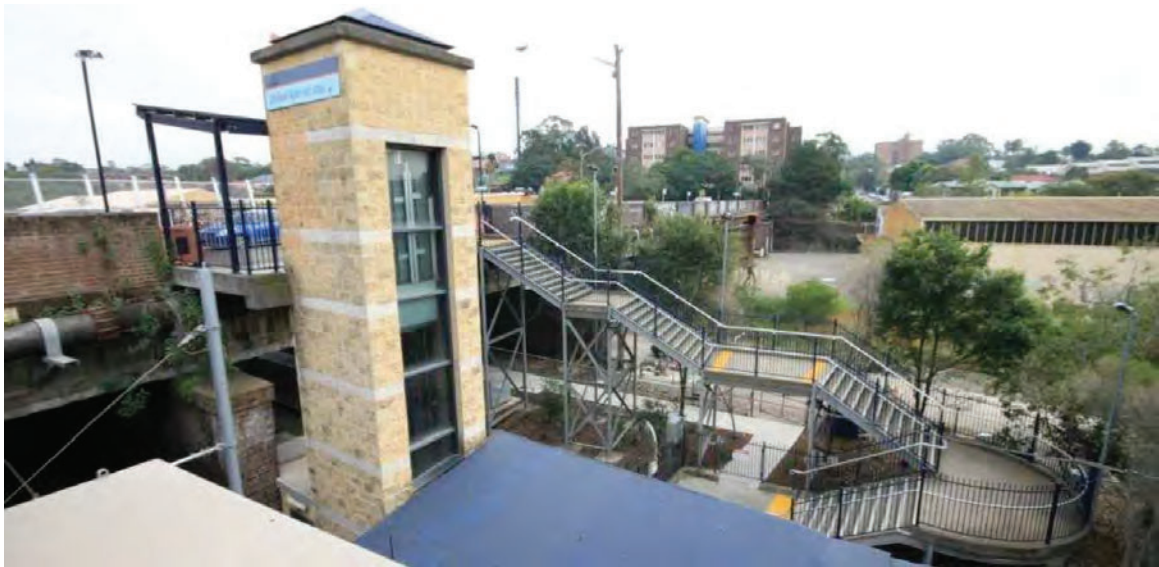
Figure 3: Photo of Lilyfield Light Rail Station
