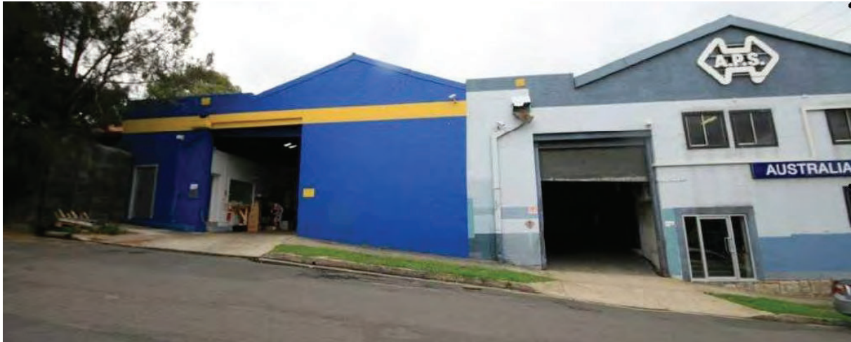
Figure 7: Photo of 36 Lonsdale Street, Lilyfield
