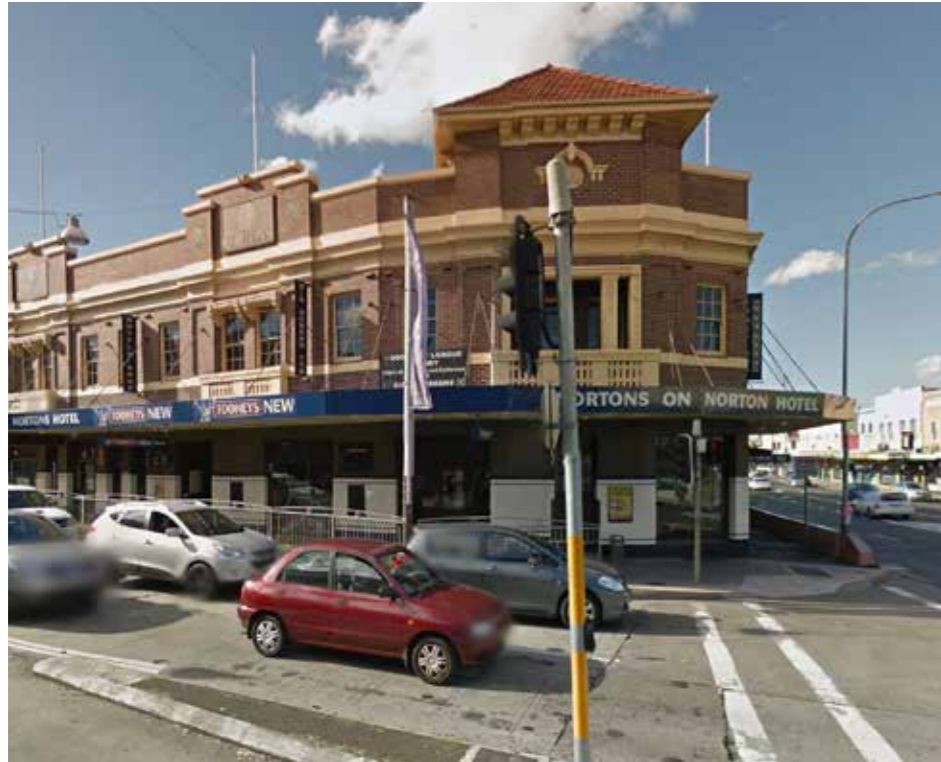
A strong heritage building marks the corner of Norton Street and Parramatta Road.
