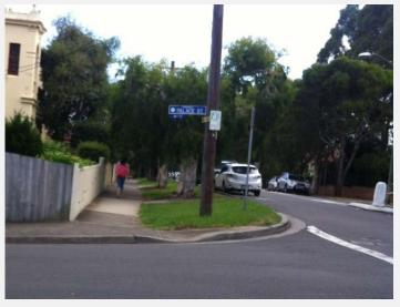
Figure 4-9: Hawthorne Pde / Tressider Ave Intersection – Missing Pram Ramp
