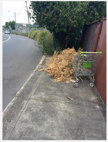
There were a number of locations throughout the study area where the footpath was identified as uneven or cracked. The footpath is generally uneven due to poor integration with manholes or poor repair after servicing. Cracks, cavities and uneven footpaths also appear due to wear, poor drainage and nearby tree roots. Adequate measures to treat footpath deficiencies are being carried by Council under its Accelerated Footpath Repair Program and are therefore not included in this study.
