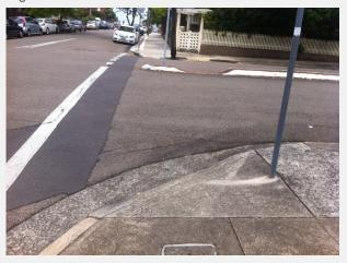
Figure 4-8: Holden St / Palace St Intersection (North-west Corner) - Non-Standard Ramp
