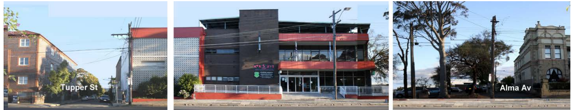
Existing Buildings Facing Stanmore Road
