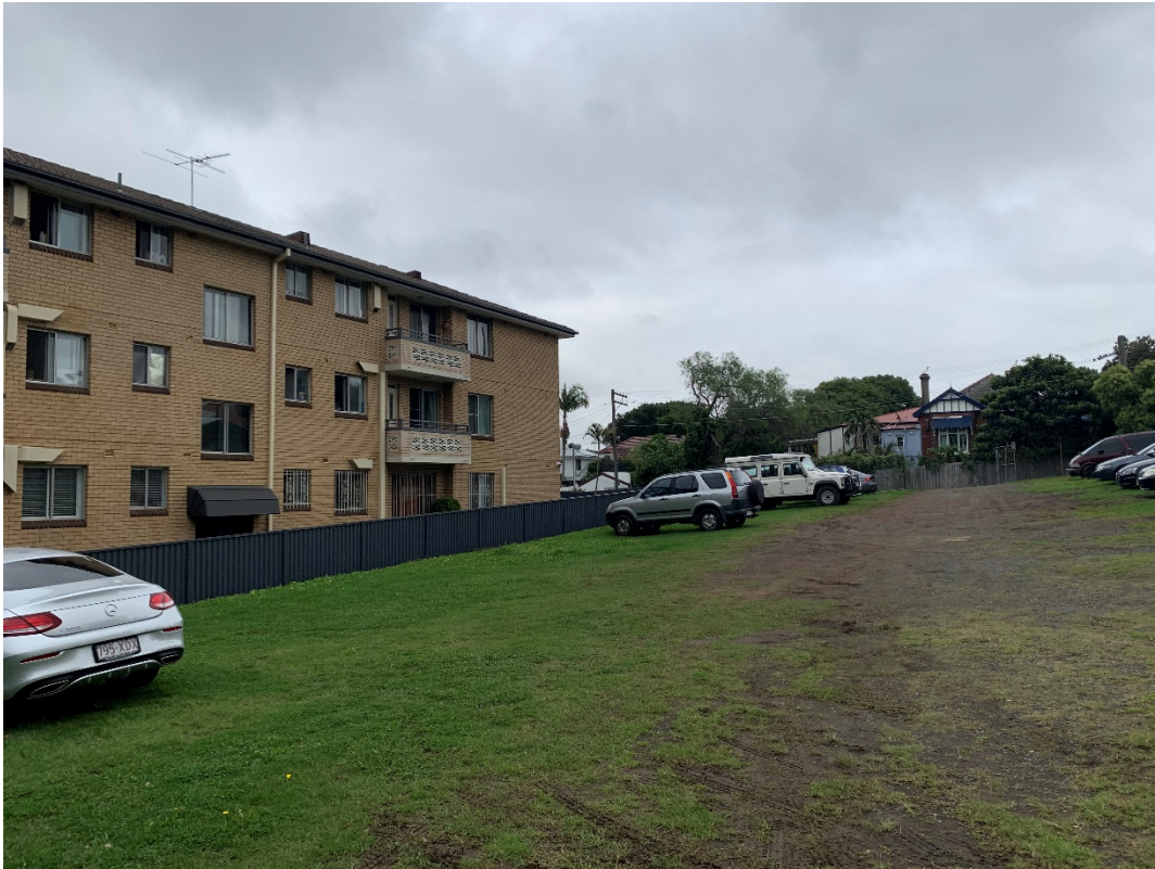
Figure 9: View of southern boundary of Site looking southwest (Source: Keylan)
