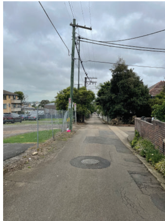
View south down Alma Avenue, mid-way down.
